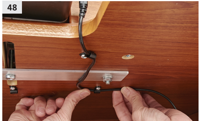
Continue to guide the foot control cord through the back cord clip. Cord may be positioned to the left or right.
