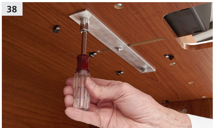
38 Secure the front base mounting bracket (K) by tightening both the base mounting bracket bolts (J) with the nut driver (Q).
